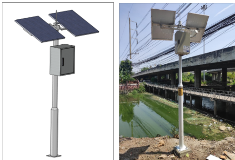
Figure 15: pLitter CCTV at Bangkok, Thailand
